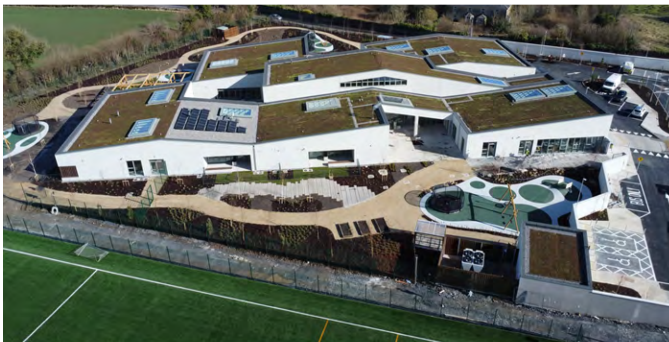
Exchequer Funded Schools Programme - St. Mary's Special School, Mullingar, Co. Westmeath
